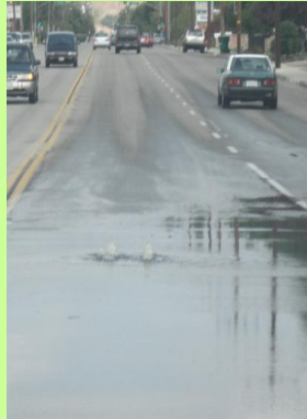
Overflowing manhole
