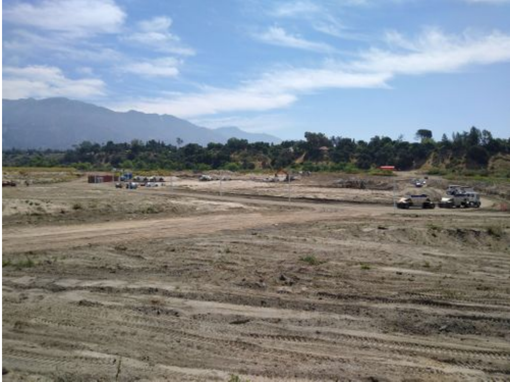
photo_1-sediment hauling operations.jpg -118.17645 34.18828
