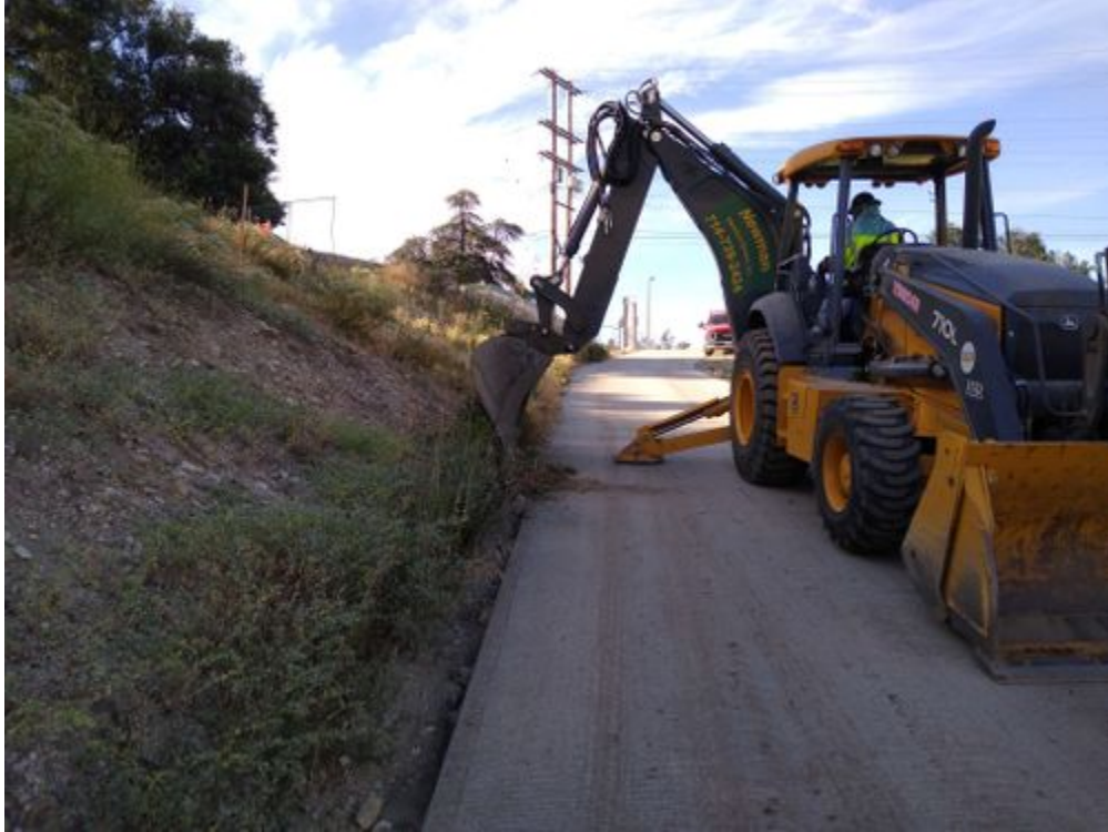
photo_1-backhoe clearing esa fenceline.jpg -118.17373 34.18584
