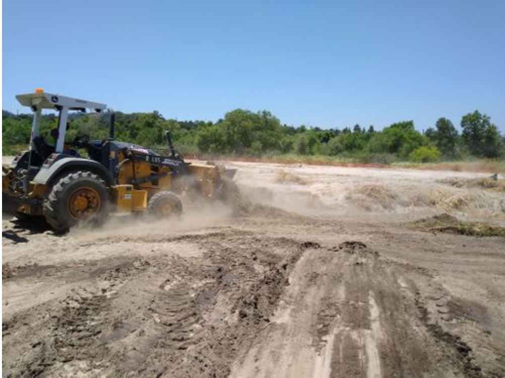
photo_3-moving vegetation stockpiles.jpg -118.17416 34.1899
