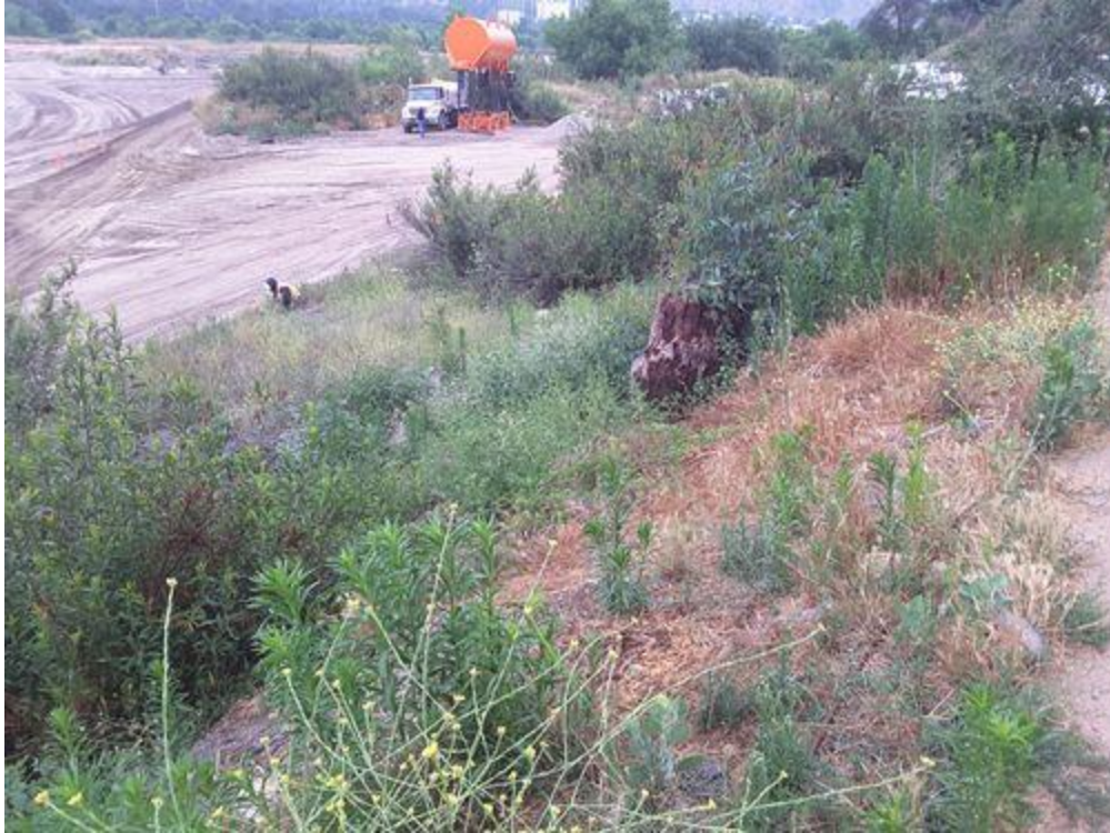
Photo 1-work area, facing N.jpg -118.17288 34.18744
