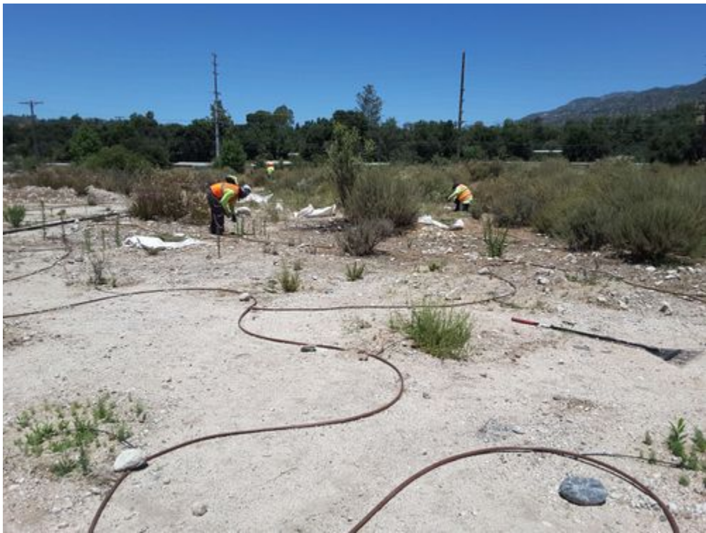
Hand-pulling in another area, facing W -118.17226 34.19501
