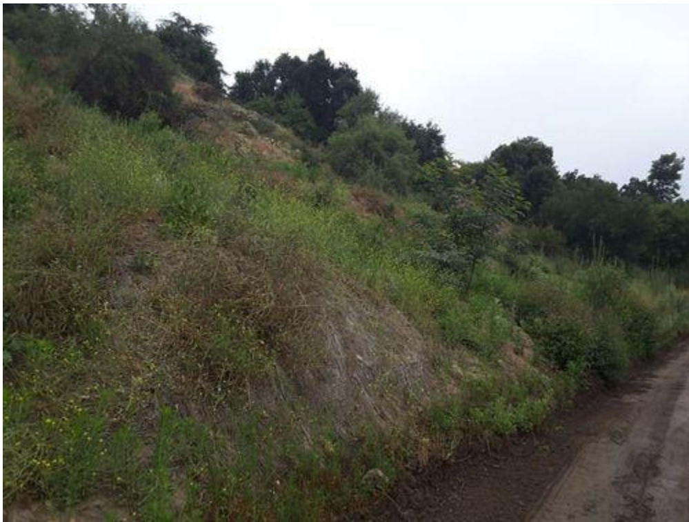
Photo 2-before hand-pulling, facing S.jpg -118.17309 34.18735
