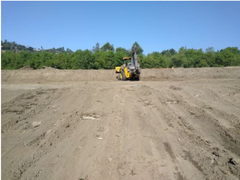
photo_2-backhoe removing vegetation.jpg -118.17594 34.1878
