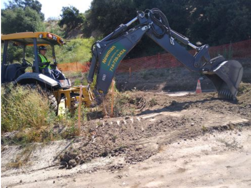
photo_3-backhoe removing vegetation at east access road.jpg -118.17377 34.18605
