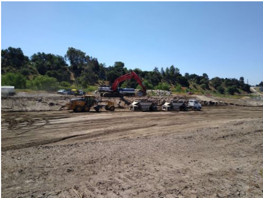
photo_2-loading haul truck.jpg -118.1736 34.1898
