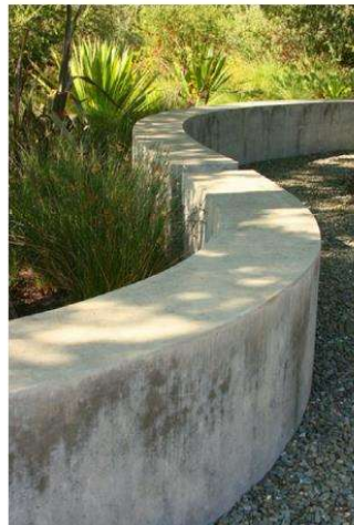
Short Retaining Wall
