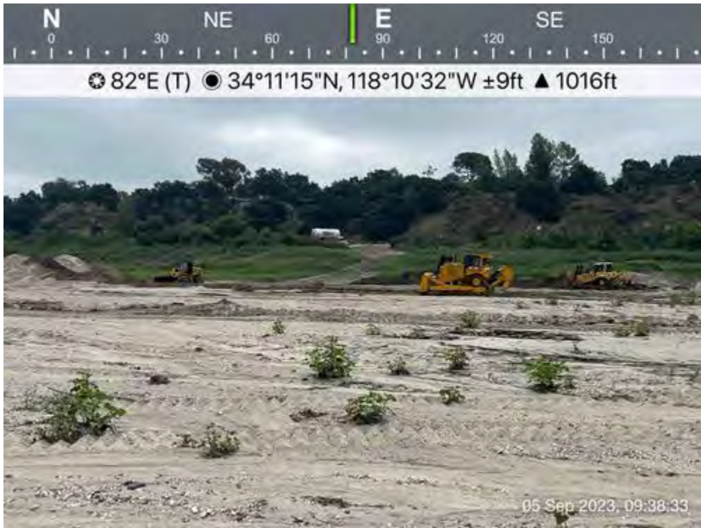
photo_2-dozers_piling_sediment_facingEast.JPG -118.17572777777778 34.18758888888888
