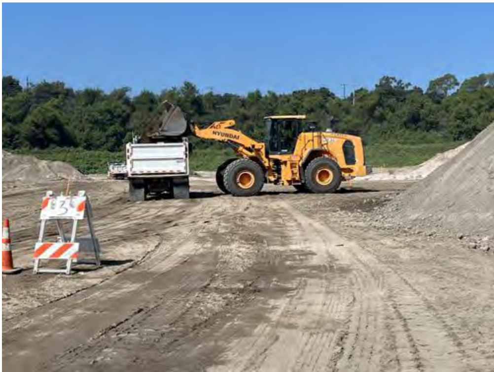
Skiploder_loading_soil_on_dumptruck_faceWest.jpg -118.17420268055557 34.18813755555555
