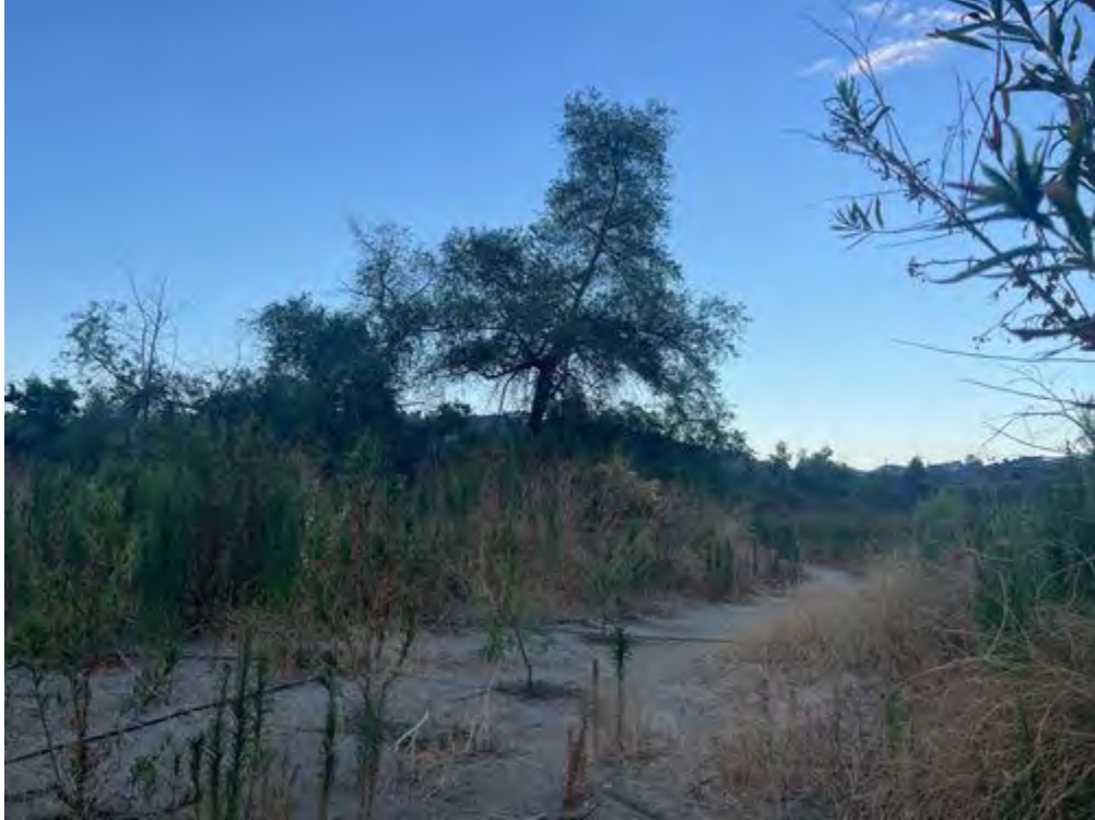
Vegetation Removal Before Facing Southwest.jpg -118.1732031777778 34.19258283333333
