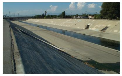
Figure 2-25. The river flows through a concrete channel for ten miles in the lower coastal plain.
