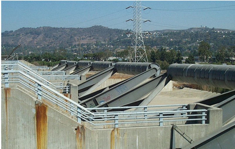
Figure 2-59. The counterweights on the spillway at Whittier Narrows Dam are significant part of this intricate structure.
