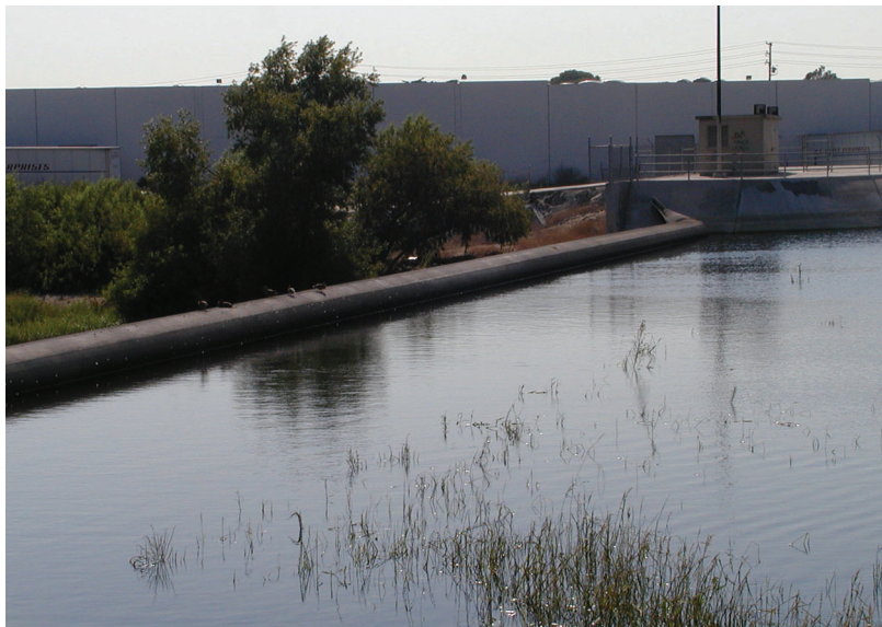
Figure 2-66. Rubber dams help the recharging process along soft-bottom stretches of the river.
