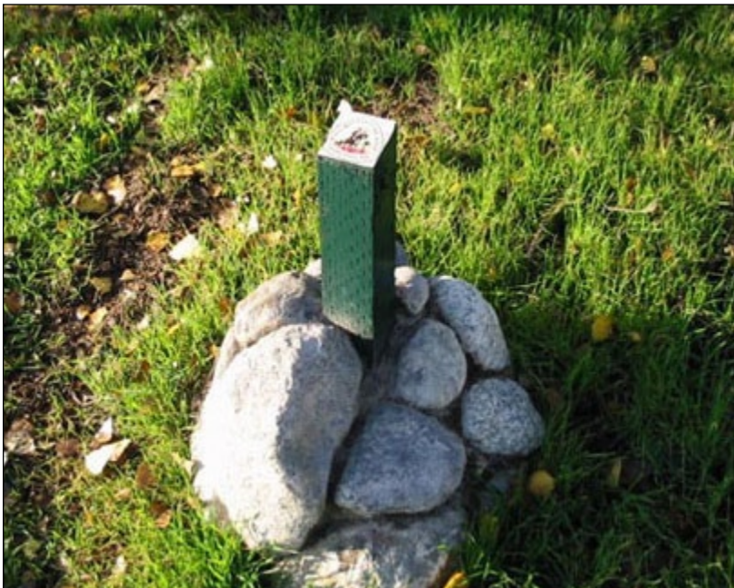
Figure 14.54 Juan Bautista de Anza National Historic Trail markers may incorporate river rock at the base along the Los Angeles River
