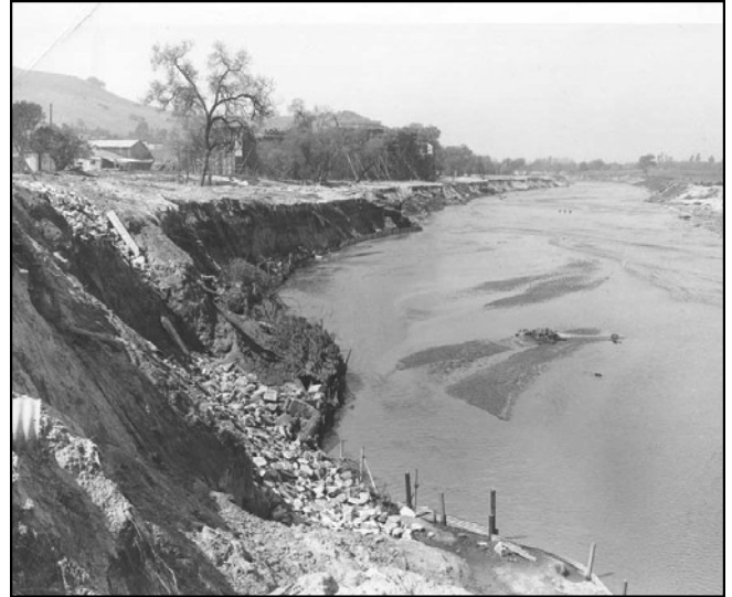
Figure A. Flood Damage in the Burbank/Studio City area, 1920s. Photo by Lakeside Golf Course Archives
