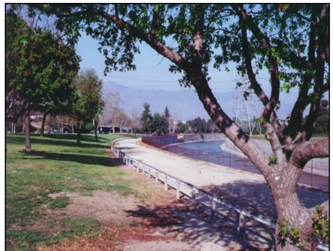
Figure B. Flood Protection Channel and multi-use trail in the Burbank/Studio City area
