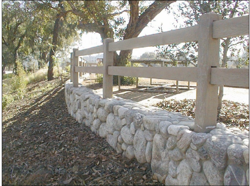
Figure 14.15 Two rail simulated wood concrete fence at Los Angeles Riverwalk installed by North East Trees and the City of Los Angeles. Installation to be done in accordance with manufacturers specifications.
