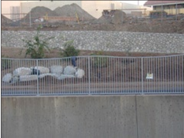
Figure 8.19 Decorative tubular steel fence along the Los Angeles River in Studio City
