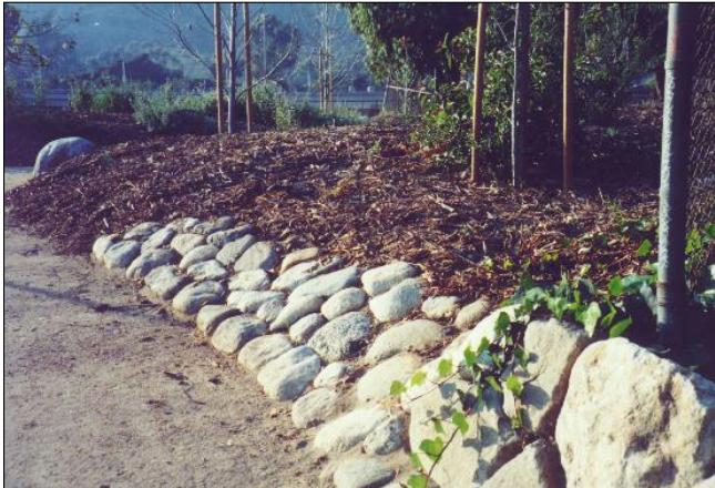
Figure 8.20 River rock edging between decomposed granite path and raised planting bed on the Los Angeles River
