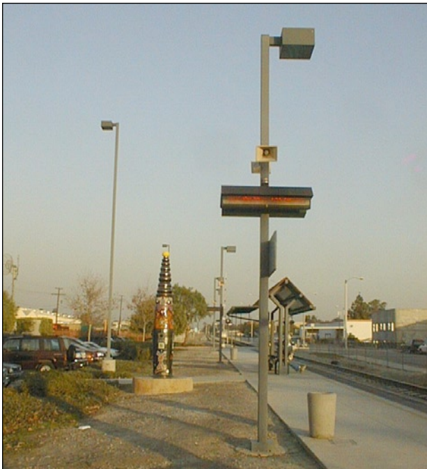
Figure 14.21 Shoebox luminaire at MetroLink Station, Pomona.
