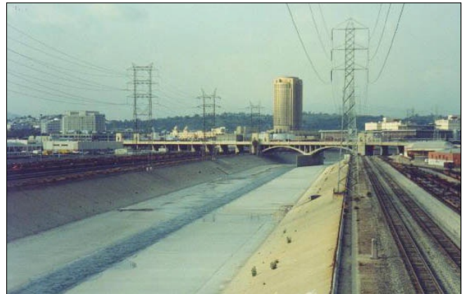
Figure 4.2 Entrenched trapezoidal condition at Fourth St. Bridge.
