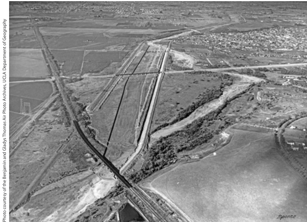
FIGURE 2.5. Levees being constructed along the Los Angeles River near Cerritos in 1932. Photograph E-3848 from Spence Air Photo collection.
