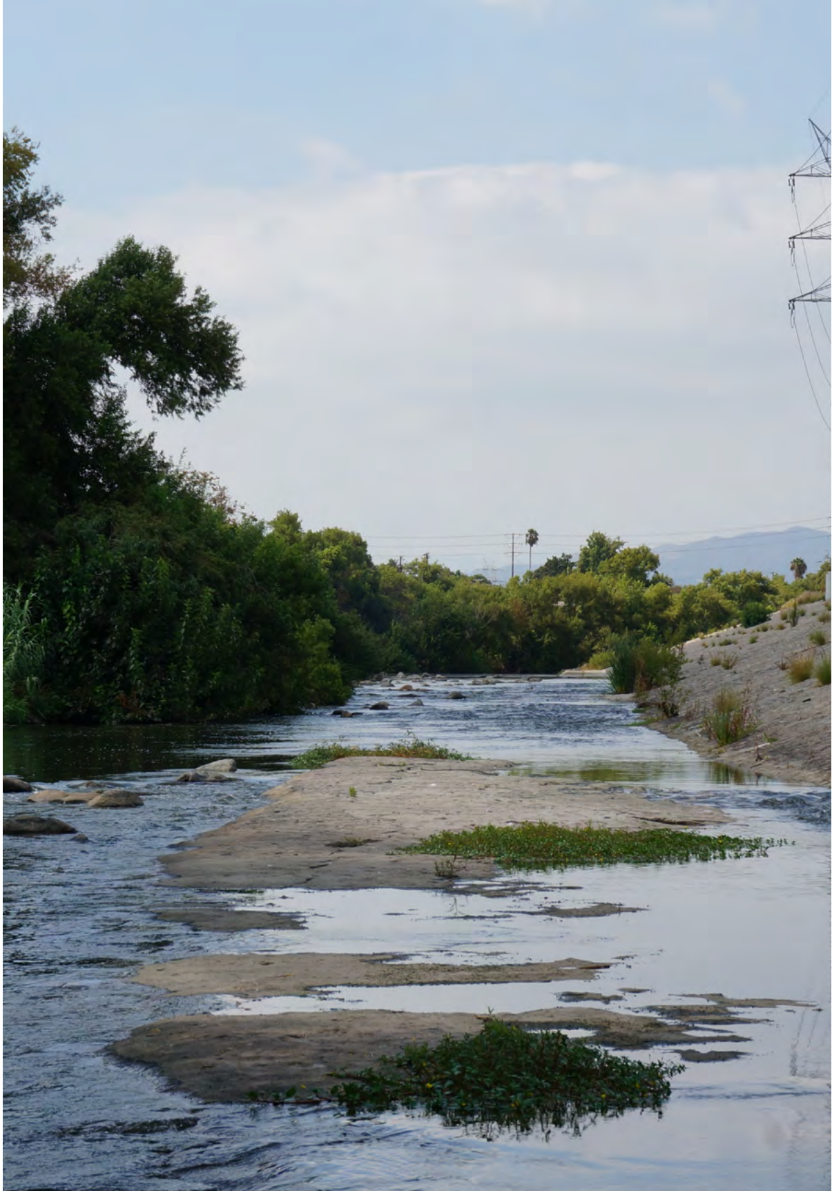
Figure 4. Certain reaches of the LA River, such as this segment near river mile 25, are soft-bottom rather than concrete. Source: OLIN, 2018.
