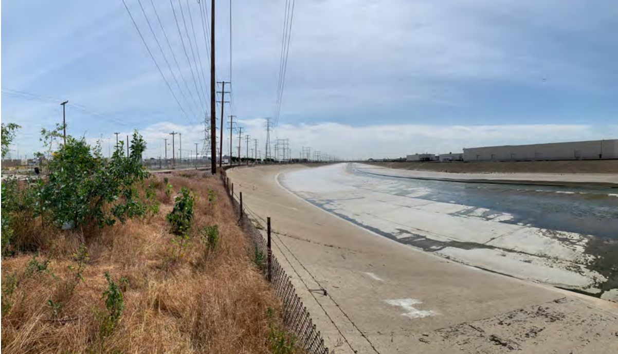
Figure 13. The industrial land that hems in the LA River, such as this example at river mile 18, is representative of over 10% of all land within the river corridor. Source: OLIN, 2018.
