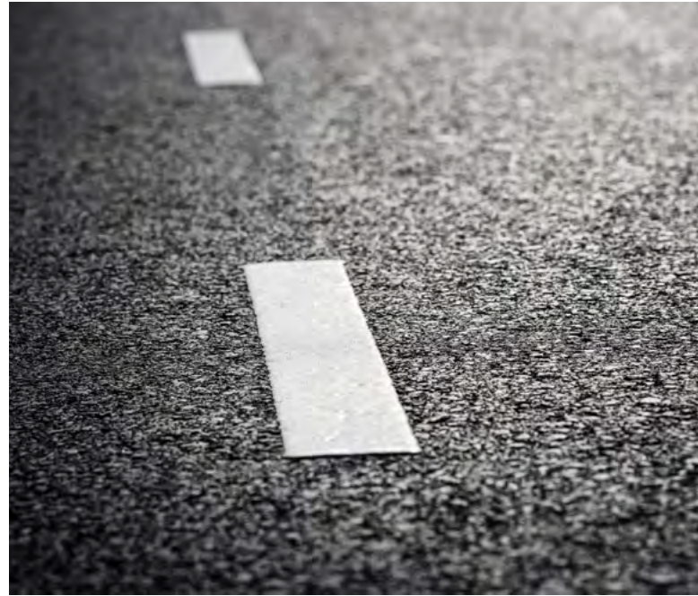
Figure 122. Thermoplastic paint is a durable option for River Mile Pavement Markings on asphalt. Source: LeManna, 2020.
