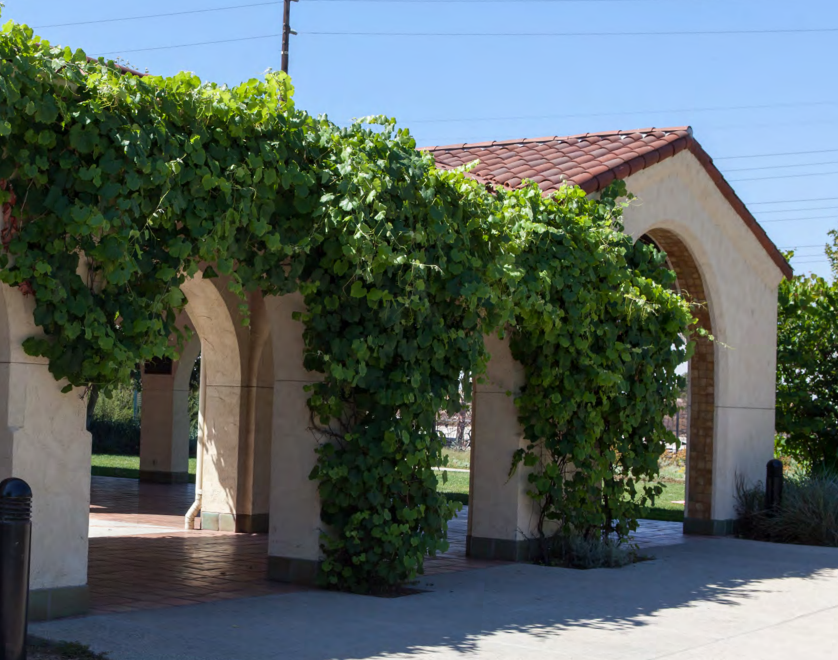
Figure 300. Lewis MacAdams Riverfront Park is one example of an existing pavilion along the LA River at river mile 26. Source: LA Public Works, 2018.
