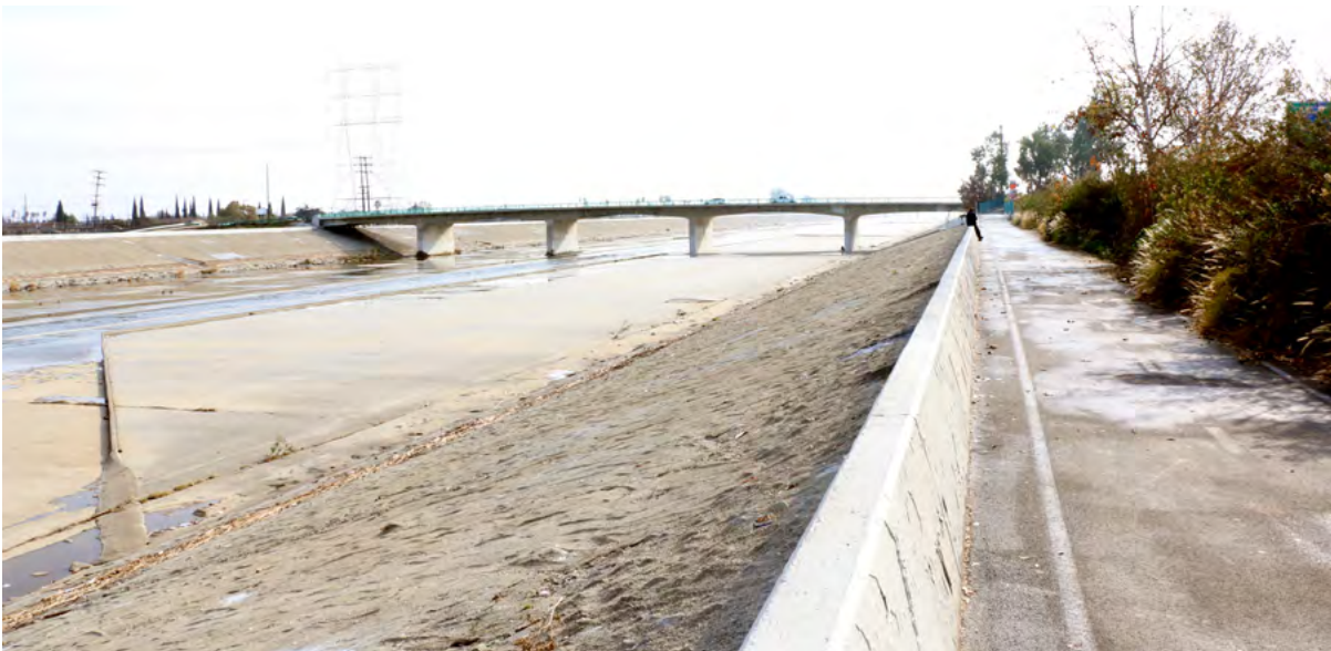
Figure 5. Certain reaches of the river, such as this segment at river mile 14, are entrenched rather than leveed. Source: OLIN, 2018.
