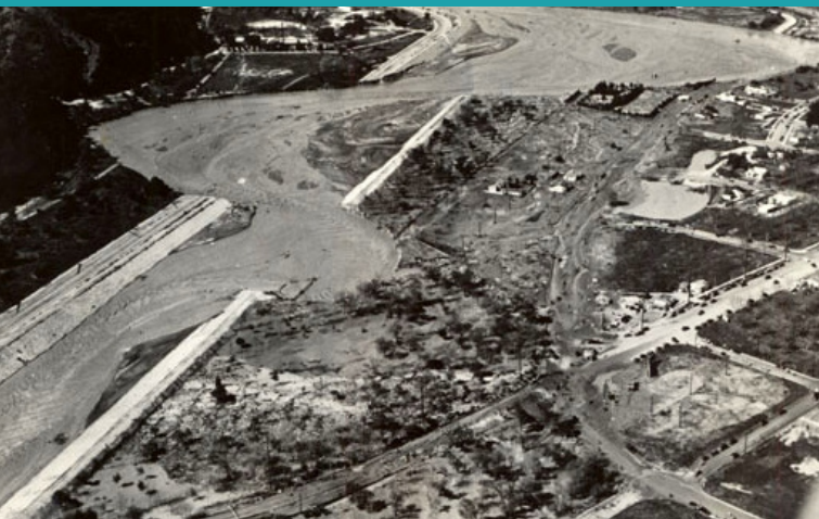
This aerial view of the 1938 flood from above Victory Blvd shows breaches in paved levees in and below a sharp curve in channel alignment. Source: USACE, 1938.
