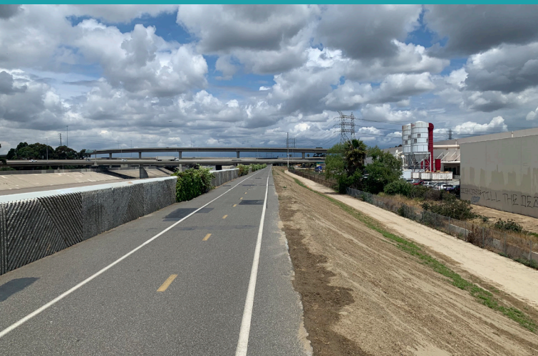
The lower river's parapet walls, such as these shown at river mile 10.1, were installed in the late 1990s in order to increase the channel capacity to greater than the 1% event. Source: OLIN, 2019.
