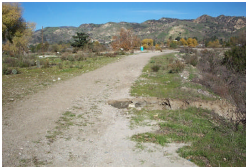
Figure 8-3b: Erosion gully near the upland area.
