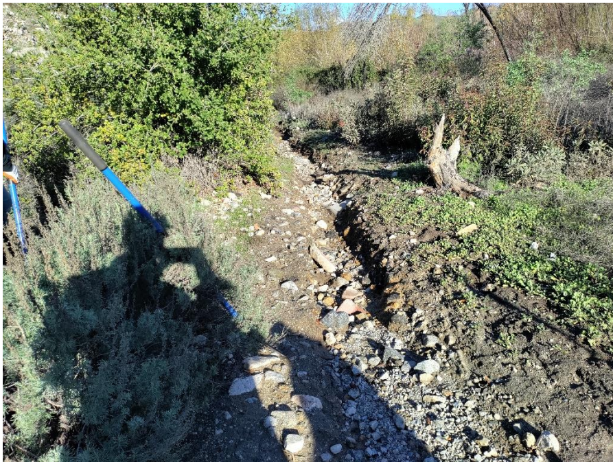
Photo 4: Area of the trail where erosion and the deposition of cobble and debris created hazardous conditions for trail users on January 17, 2023.
