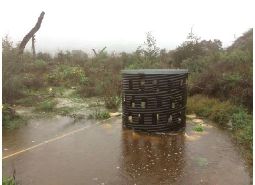
**January 2019.** An outlet tower at the center of the spiraling drainages conveys storm flows from the deck of the SPS into the Santa Anita Channel (to the west) via an underground pipe. This photograph was taken during a heavy rain event, and it shows the proper/unobstructed flows into the outlet tower.
