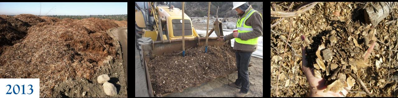
Here are some of the stockpiled natural materials. Whatever trunks/stems were not retained whole, were mulched for use in conditioning the placed sediment. We essentially used 'the whole animal' in terms of woody vegetation from the Middle SPS.
