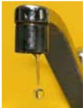
Leaky faucets are a common cause of water waste and are very easy and inexpensive to repair. A dripping faucet can waste up to 2,700 gallons per year, which will add to the cost of your water and sewer bills. You can easily repair dripping faucets by replacing washers available at your local hardware store.
